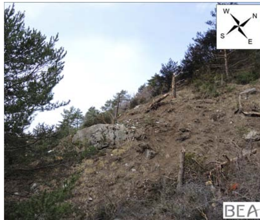
Figure 13 - contact area with vegetation
