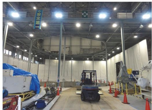
Fig. 9 Vacancy after the demolition. Piles were left in the ground.
