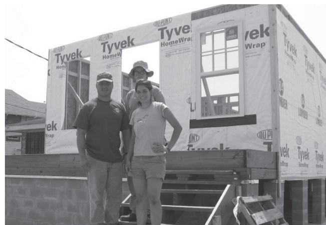
**BEFORE AND AFTER**--This is the house we worked on most of the day. The Tyvek was completed and chalk lines placed for the siding; Staples were hammered down; closets framed; flooring was leveled; and the yard was graded. On the right are our supervisors Emily and John.
